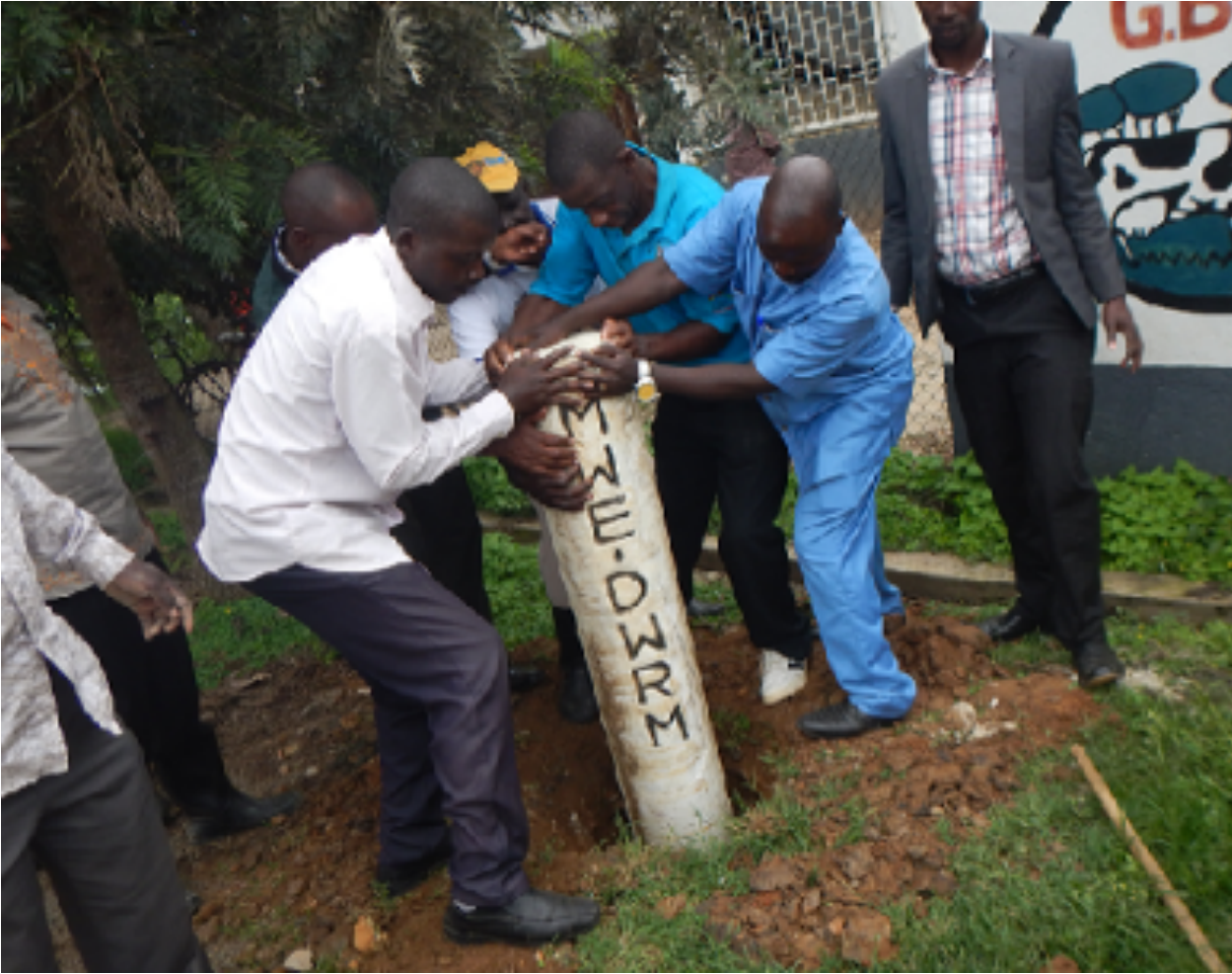
Plate 10: Installing a boundary pillar near GBK premises
