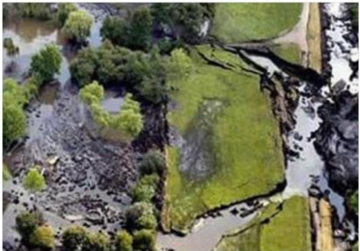
Levee breakthrough (drought)
