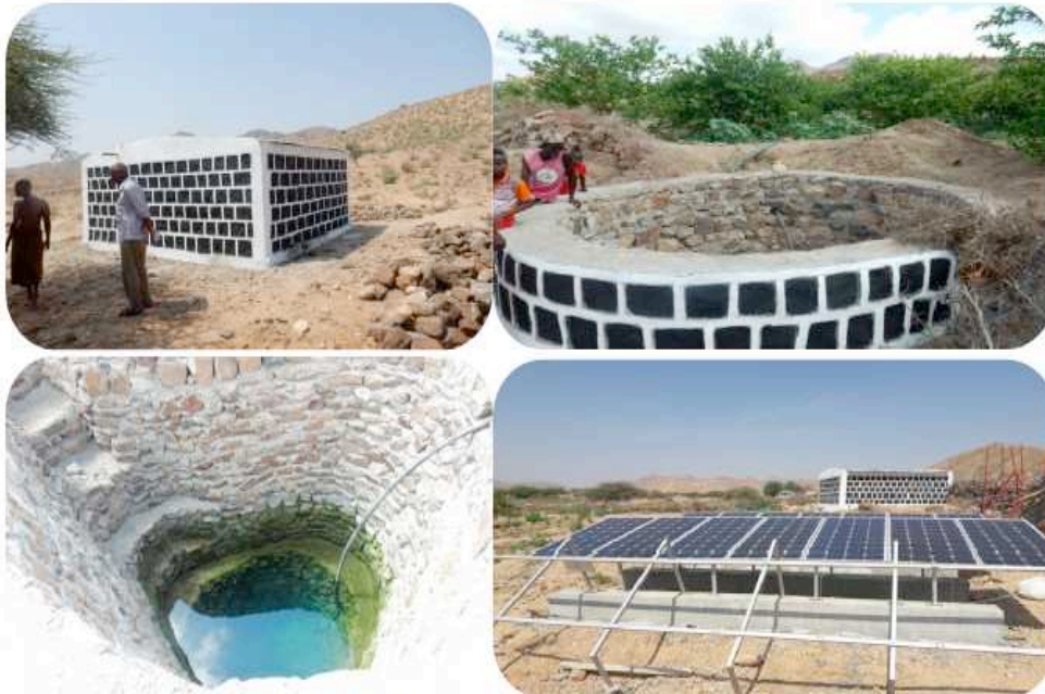
Water wells and water storage facility equipped with solar pumps, Assamo Landscape, Djibouti
