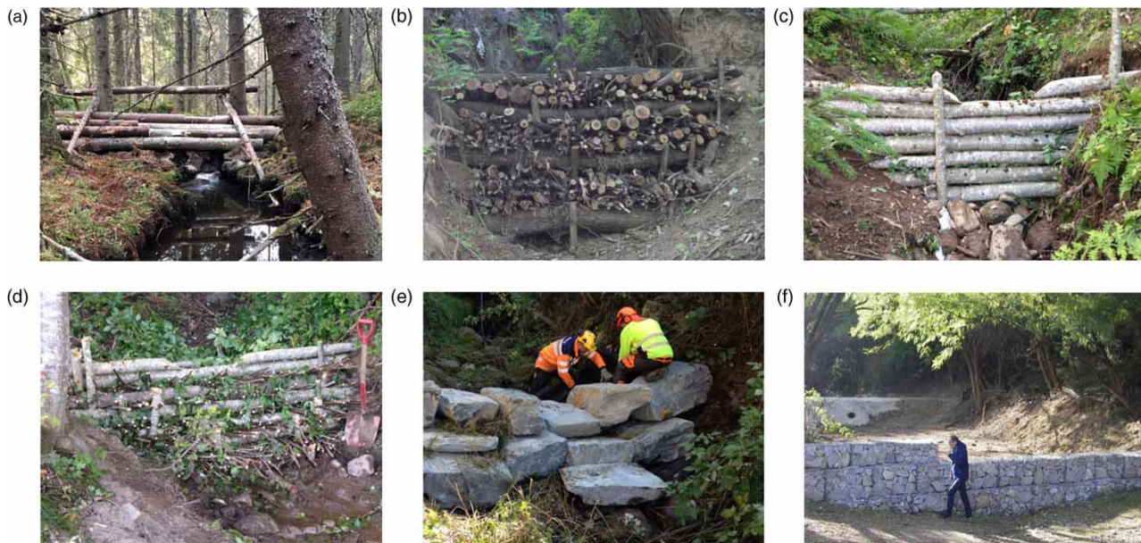
Figure 1 | Examples of online Natural Flood Detention Facilities including (a) leaky woody dam, (b) brushwood dam, (c) log dam, (d) log and branch dam (d), (e) stone check dam, (f) gabion dam. Dams a, c, d and e are made in Norway, b and f in Slovakia. Photo (e): S. Myrabø.
