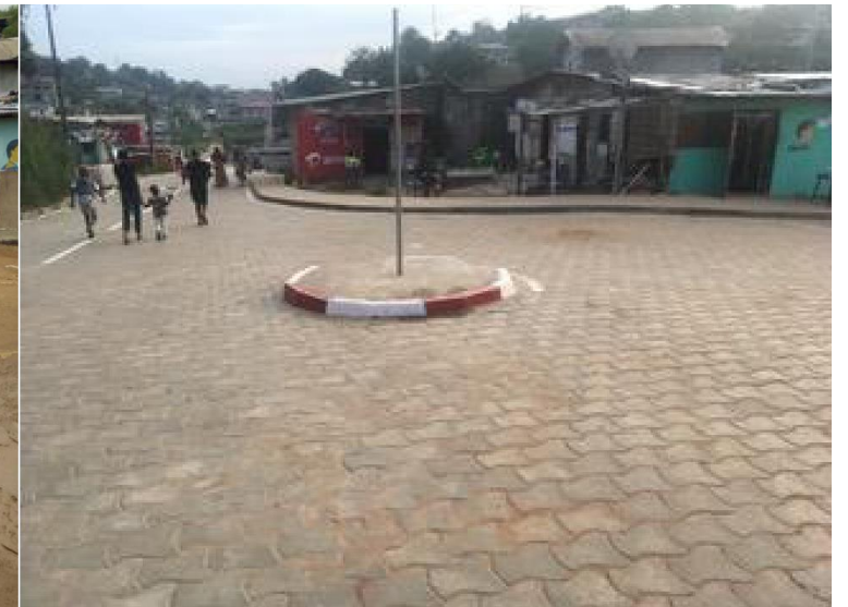
State of the environment after the work is carried out
