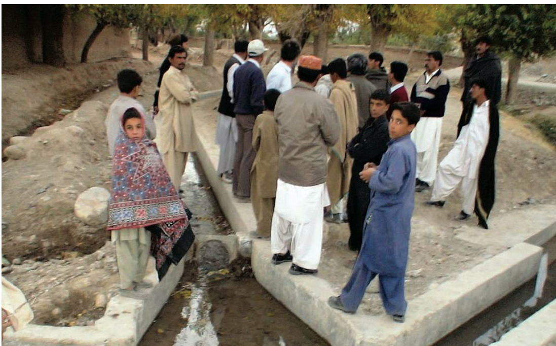
Lined water conveyance channel taking water to irrigation fields from the rejuvenated Karez after successful artificial recharge © Salman Ali
