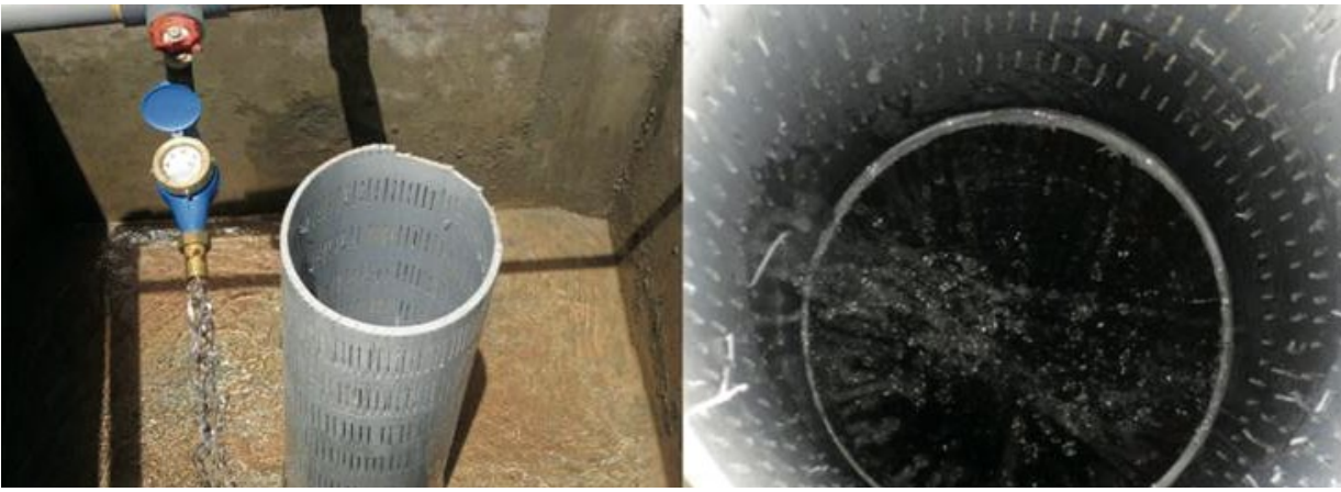
The recharge mechanism. See the water brought in from dam gushing in the ground through slotted pipe after filtration © Dr. Abdul Majeed
